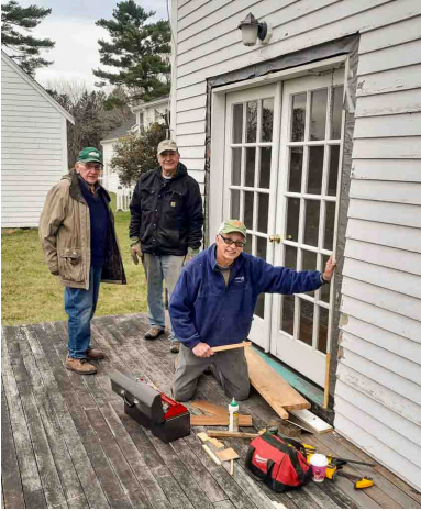
Bruce, Jerry and Ian replacing the door trim
